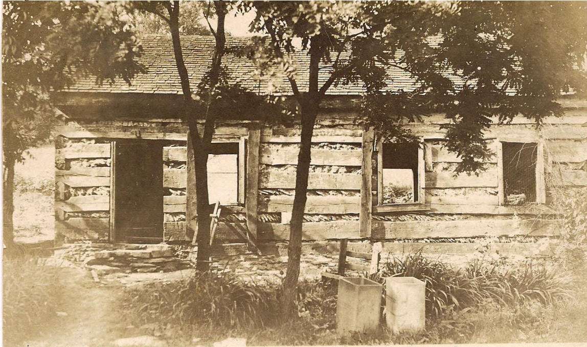
This earliest photo of the cabin shows the solid logs, the missing chinking, and the absence of doors and windows.
