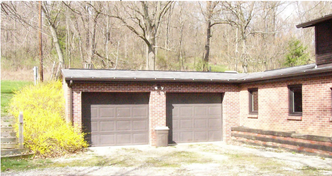
Our addition included a two-car garage, a second bath, and additional storage.
